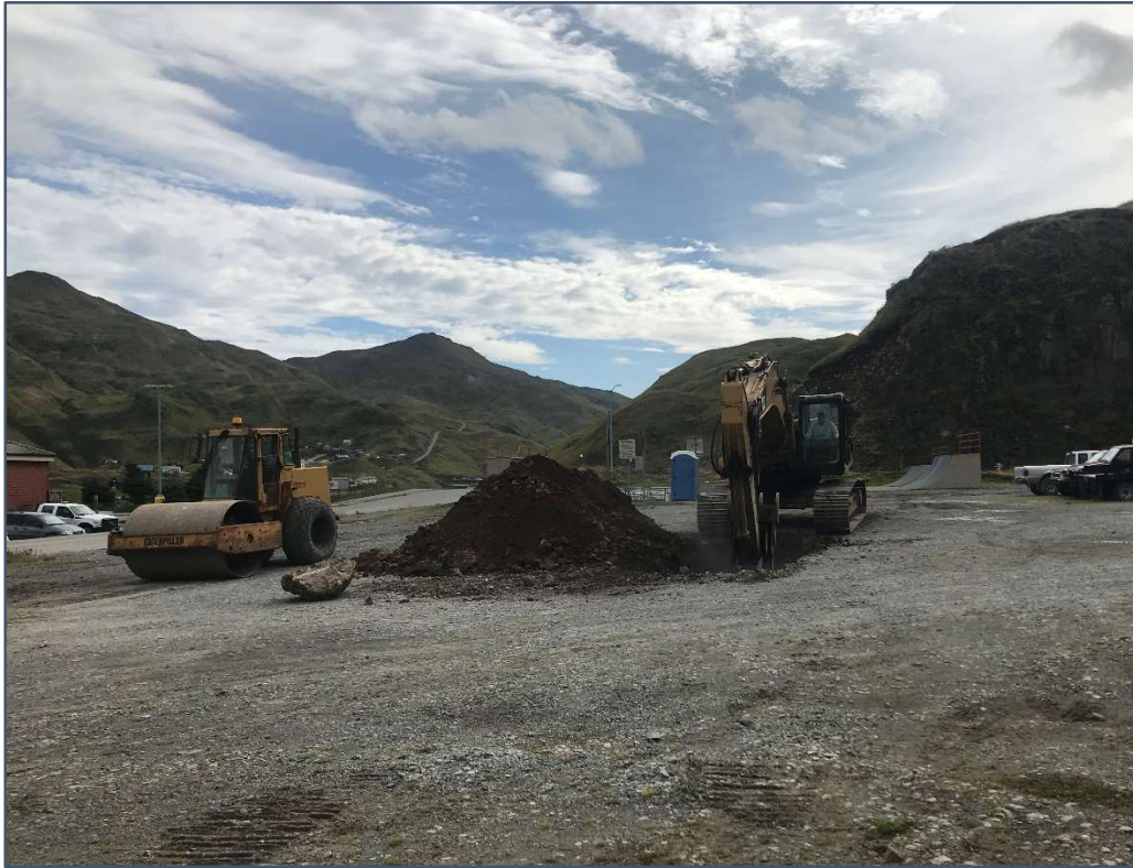
Figure 2-4. Test Pit Excavation
